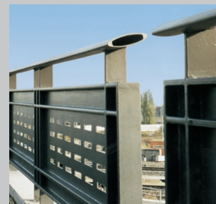
Special profiles for handrails on bridges
